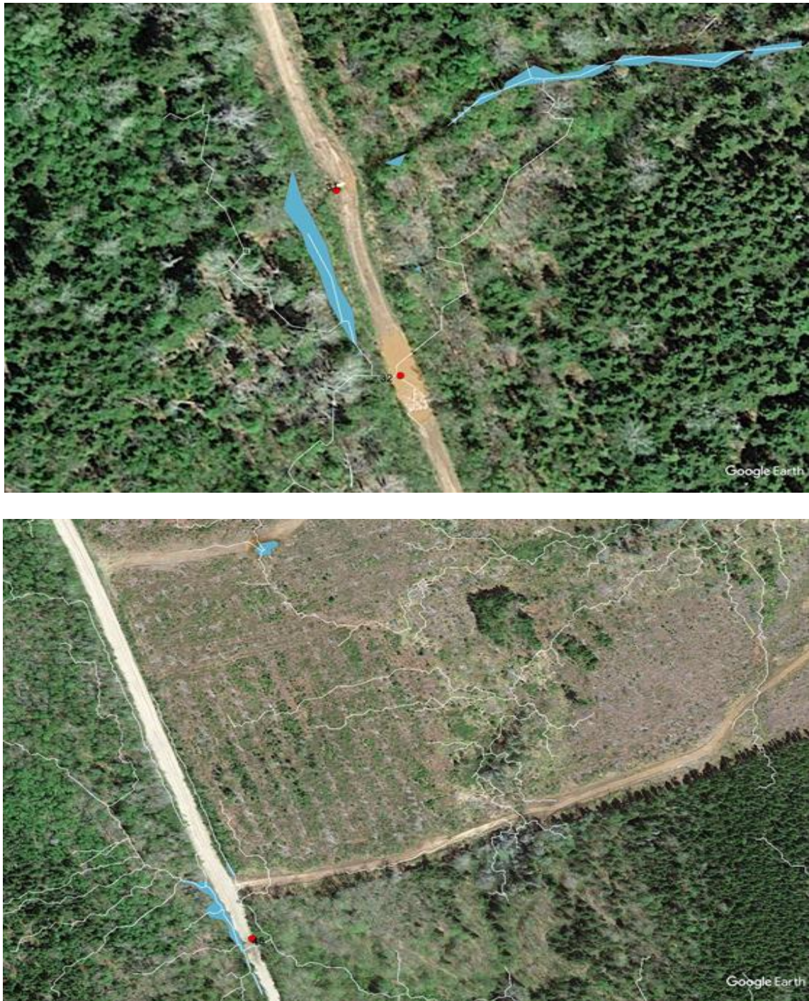
Figure 5.4. Road deterioration examples along the Aboujagane road segment: road braiding with partial culvert exposure and flooding at Location 31, and flow-induced road flooding at Location 32 (top); flow-induced road flooding at Location 32 LiDAR-derived flow channels: white lines; flow induced road narrowing at Location 45 (bottom). LiDAR-derived flow channels: white lines; depressions: blue polygons.
