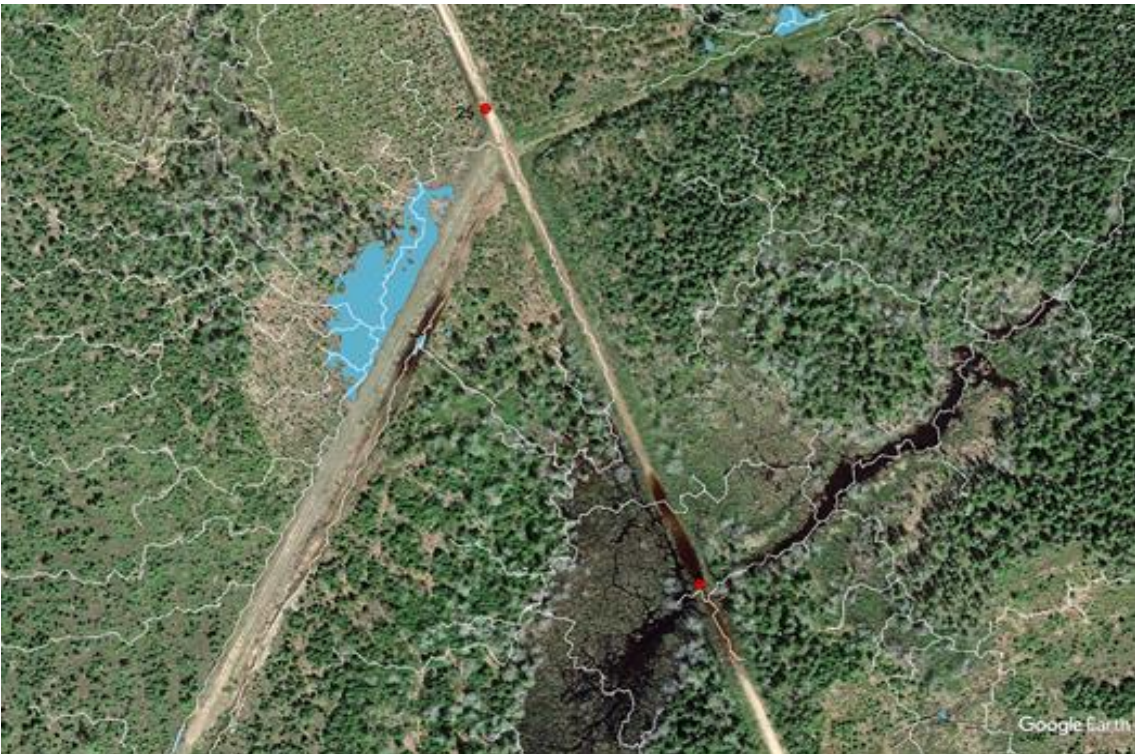
Figure 5.3. Road deterioration examples along the Aboujagane road segment: hydro-network channel induced flooding at Locations 29 and 30 (top); wetland-induced flooding at Location 26 coupled with channel-induced water flow along the road at Location 25. LiDAR-derived flow channels: white lines; depressions: blue polygons.
